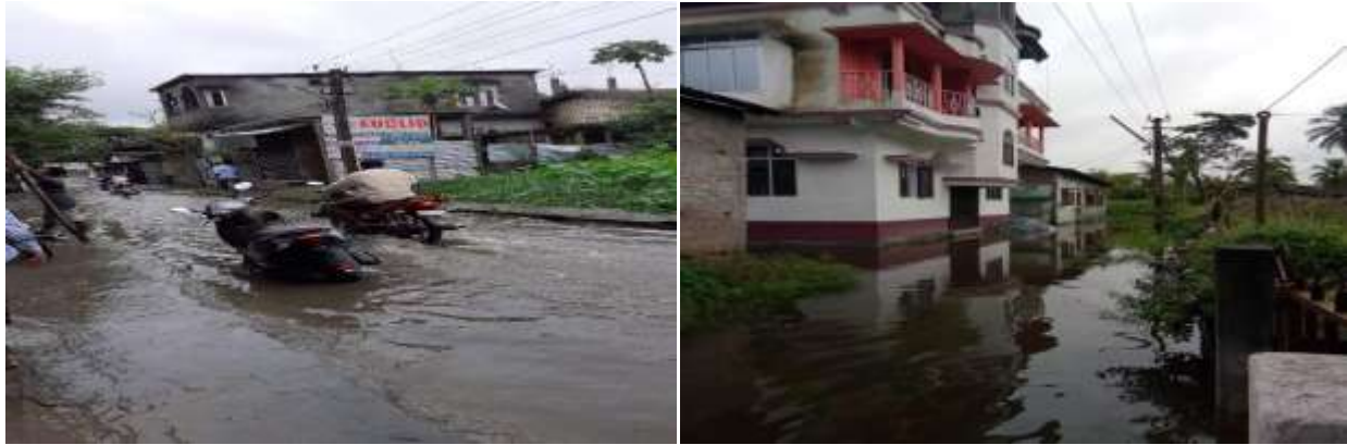
Fig- 7: Effects of Poor drainage
