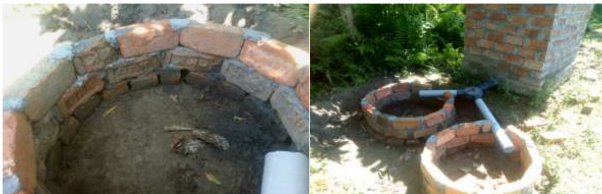
Fig- 4: Poor construction of IHHL
